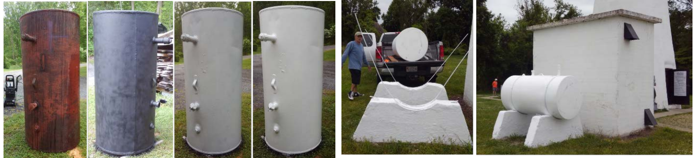
Power washing rust off
